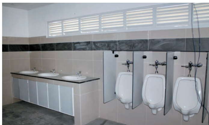
Upgrading of CAS Second Floor Comfort Rooms (93% completed)
