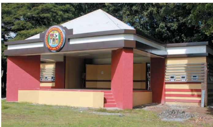
Improvement of Center Stage (100% completed)
