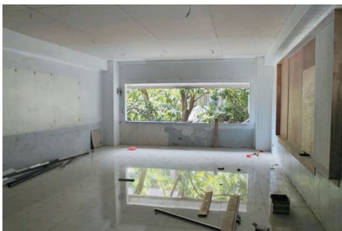
Construction/Expansion/Rehabilitation of Academic Bldg. CAS Classroom 3, 4, 5 & AVR (95% completed)
