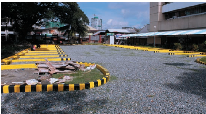
Construction of Parking Spaces in Obrero Campus (100% completed)
