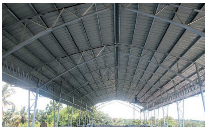
Construction of Roof of Academic Building at Mintal Campus (100% completed)
