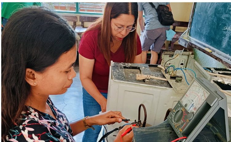
Women Empowerment: Two female participants check the electrical components of an air conditioning unit during the DomRAC Troubleshooting and Repair activity.
